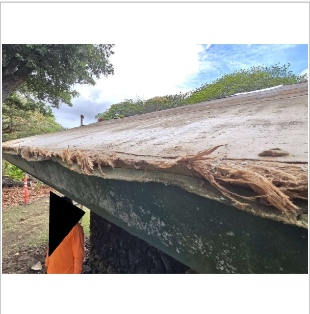
Waianapanapa State Park_Comfort Station Reroof_T&G Roof Decking in poor condition.
